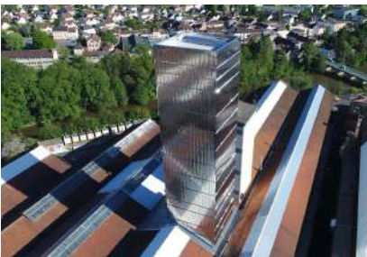
Gueugnon (France) Cold-rolling mill and finishing facilities
