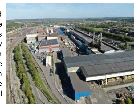
Photovoltaic panels on Châtelet roofs.
