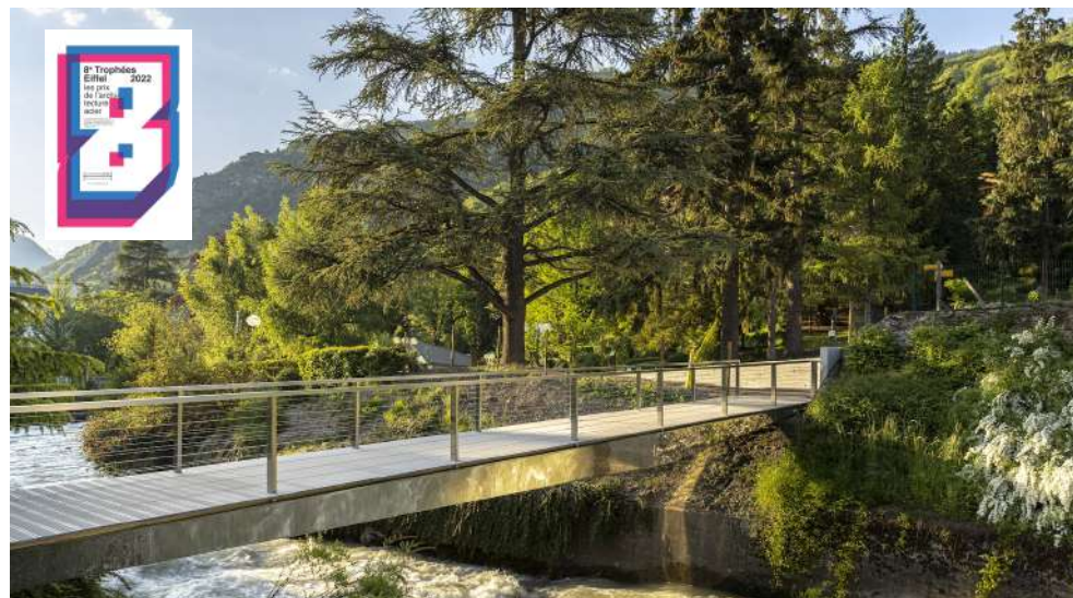
The girders of the Brides les Bains footbridge are made of Aperam 304L stainless steel, with a Uginox polished mirror reflecting the eddies and movements of the water. The footbridge thus changes with the seasons and the weather, and allows for discrete integration into this alpine environment.
