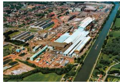
Isbergues (France) Cold-rolling mill and finishing + Recyco
