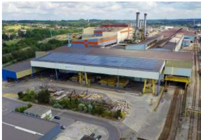
Châtelet (Belgium) Melt shop and hot-rolling mill
