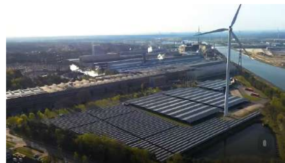
Windmill and photovoltaic panels at the Genk (including the parking area).
