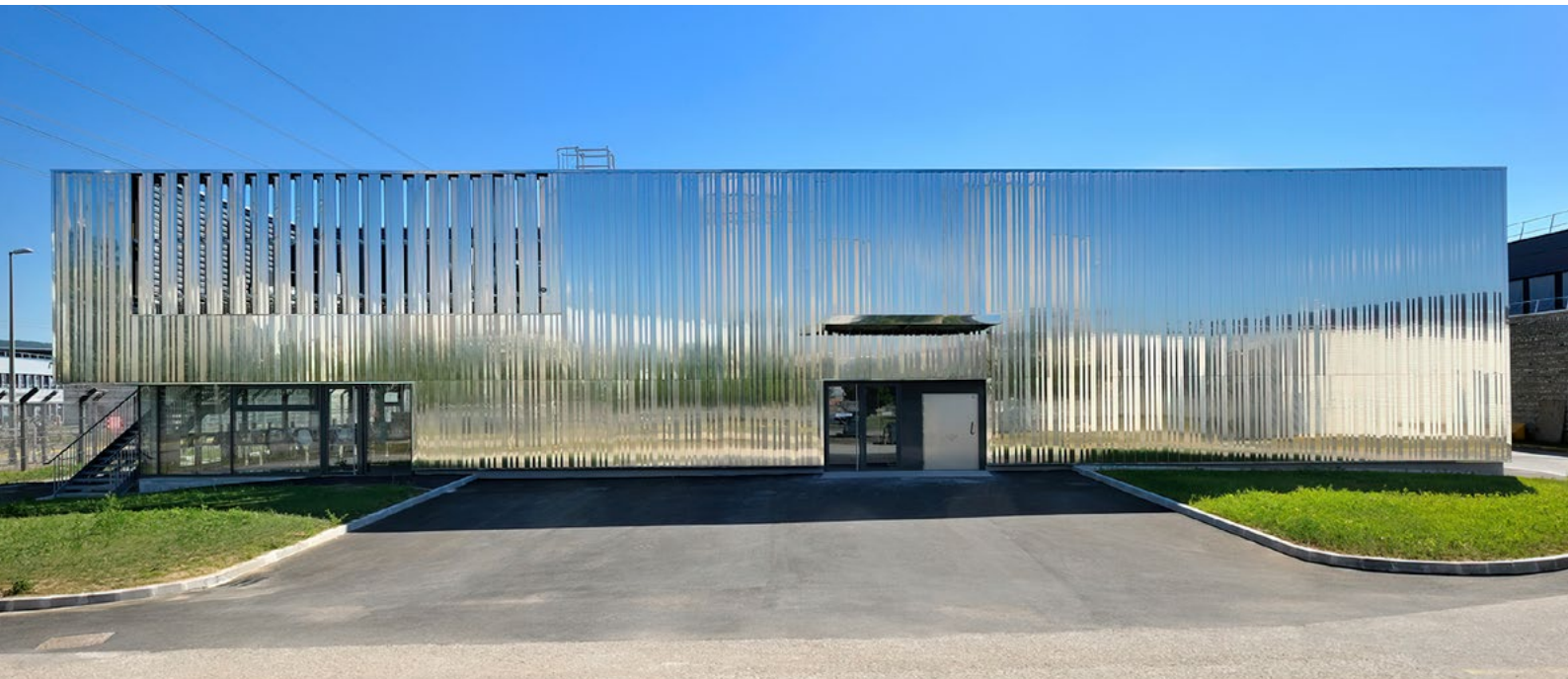
Student restaurant EDF/UFPI campus | Saint-Vulbas, France | SOHO ATLAS IN FINE © Vincent Ramet | Aperam 304L, Uginox Bright
