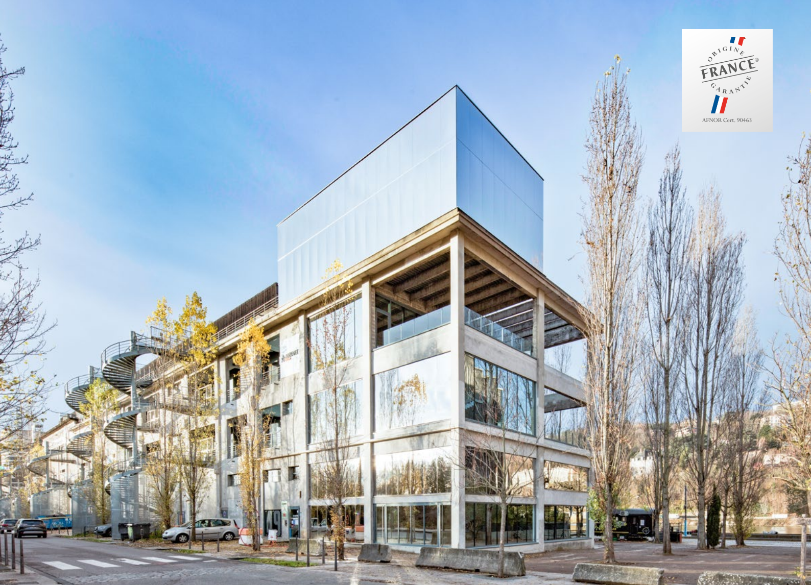
Rehabilitation of the pergola of the Sucrière | Lyon Confluence, France | Z ARCHITECTURE © Jonathan Letoublon | Aperam 304L, Uginox MECA 8 ND®.
